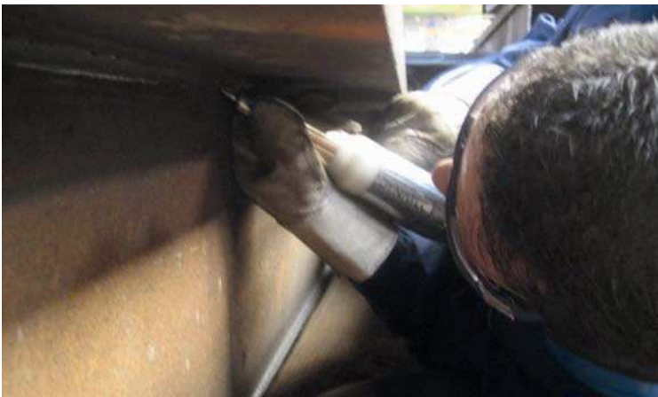
Figure 7-3: Post-weld treatment of fillet welds on the Schenkendorfstraße Bridge
