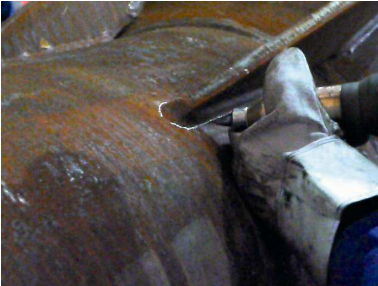
Figure 7-7: Post-weld treatment on vibrating heads, Schachtbau Nordhausen
