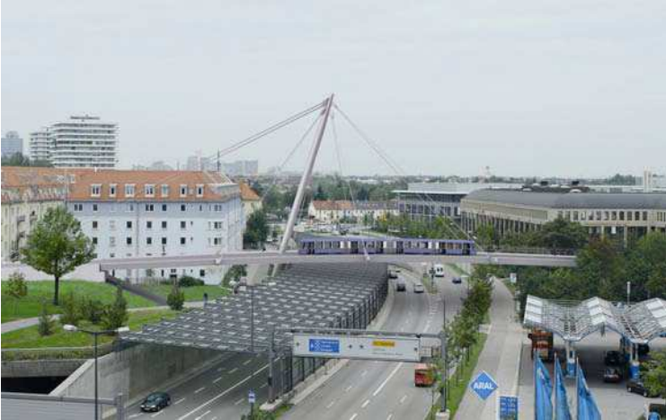
Figure 7-2: Schenkendorfstraße Bridge over the Mittlerer Ring (ring road), Munich
