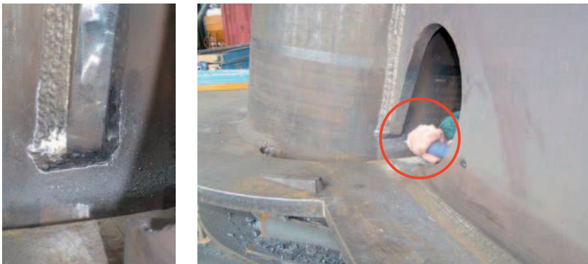
Figure 7-6: HiFIT post-weld treatment on the lower area of the transition piece.
