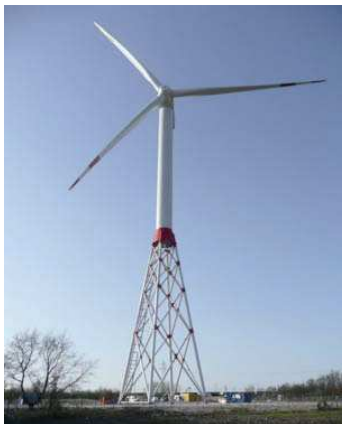
Figure 7-4: REpower wind turbines with jacket near Bremerhaven
