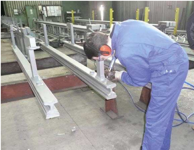
Figure 7-1: HiFIT treatment of a swivel joist, Maurer Söhne
